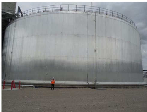
Figure 64. Left 175 : A hot storage tank at the 110 MW Crescent Dunes CSP power tower plant in Nevada holds molten salt at 565°C and can deliver 10 hours (1100 MWh) of stored solar energy at any time day or night. Right 176 : The principles of combining molten salt storage with solar power (same plant in Nevada).
