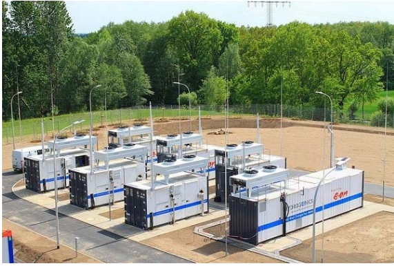
Figure 60 149 . Left: photo of the Falkenhagen P2G plant. Right: X-ray illustration of one container showing the electrolyzer stacks inside
