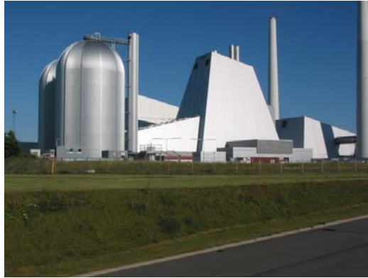
Figure 65. District heating water storage tanks (to the left) in connection with a power plant 177 .
